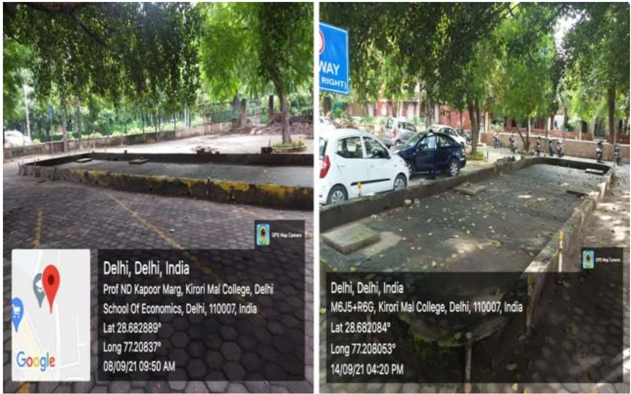
Rainwater Harvesting, Parking Area
