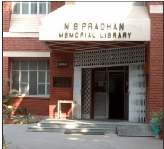
Two iron grating covers have been placed as foot mats. These can trap front wheels of a wheelchair as well as white cane and the collapsible gate's threshold poses a trip hazard for everybody.
